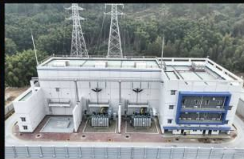
YUNFU SUBSTATION OF CHINA SOUTHERN POWER GRID
