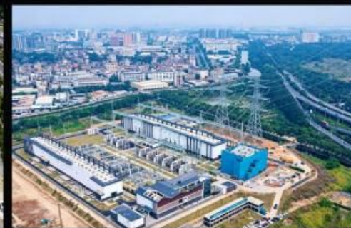
DONGGUAN SUBSTATION OF CHINA SOUTHERN POWER GRID
