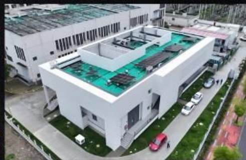
ZHUHAI SUBSTATION OF CHINA SOUTHERN POWER GRID
